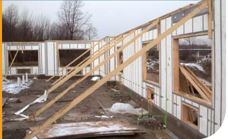
While the use of expanded polystyrene (EPS) in construction has been fueled by the residential market for decades, the incorporation of insulation system panels into commercial structures is gaining momentum. As design professionals attempt to respond to building requirements for energy efficient design, lower operating expenses and rapid construction, the engineered panelized approach creates economies of scale.
